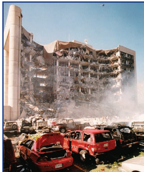
Alfred P. Murrah Federal Building, Oklahoma City 1995
