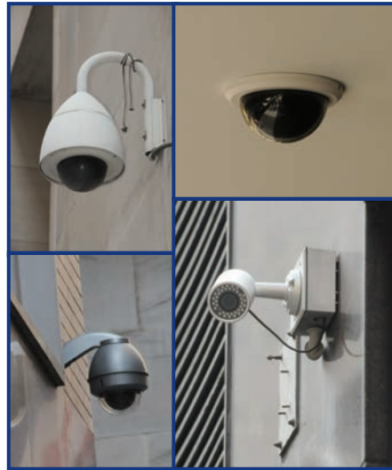
CCTV cameras in many shapes and sizes.
