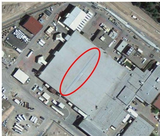
Figure 5. PF-4 Roof Showing Drag Strut Drag strut is circled
